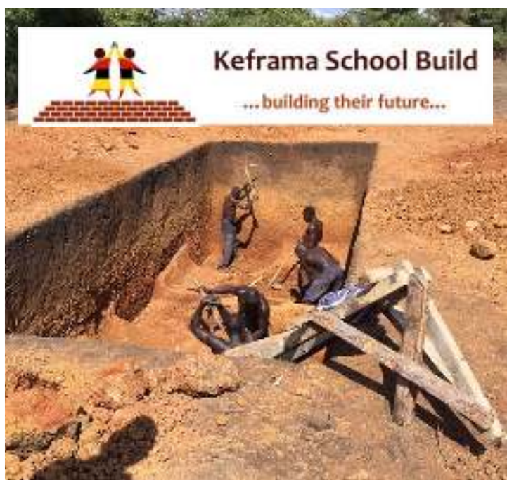
Work is under way... digging for the latrines
