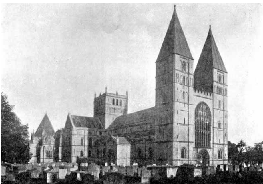
Southwell Cathedral from North-West.
